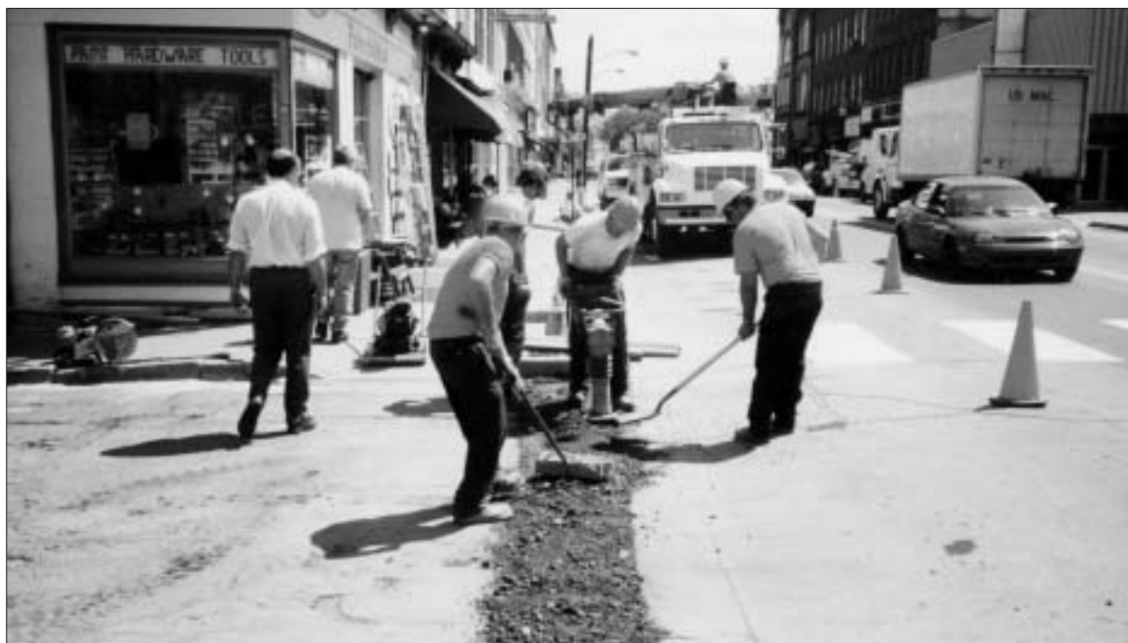
The Cornell structural soil is lightly compacted and will support the weight of concrete and asphalt.
