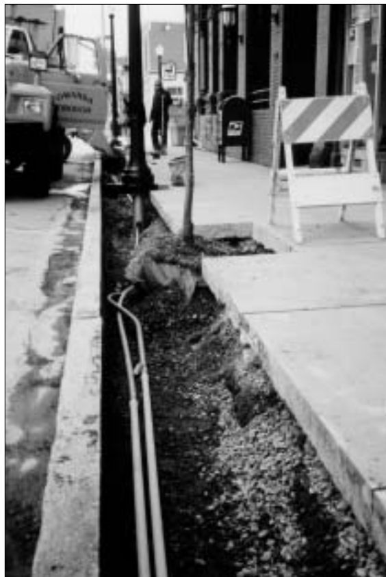
A trench is constructed for both tree roots and electric lines.
